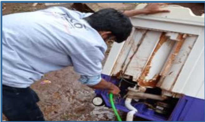
Repaired household equipments and electrical wiring of flood affected families of Chiplun and Mahad.
